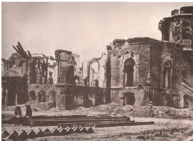
Fig. 17 – Ruins of the Residency in Lucknow
