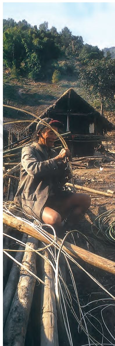
Fig. 5 – A log house being built in a village of the Nishi tribes of Arunachal Pradesh.
